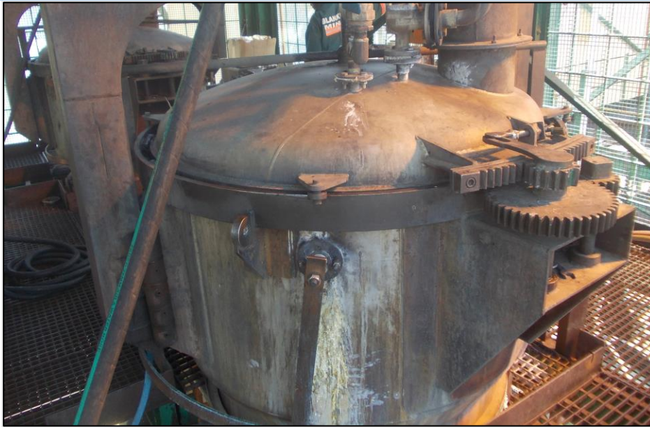
Figure 71: Elution and Electrowinning Vessels
